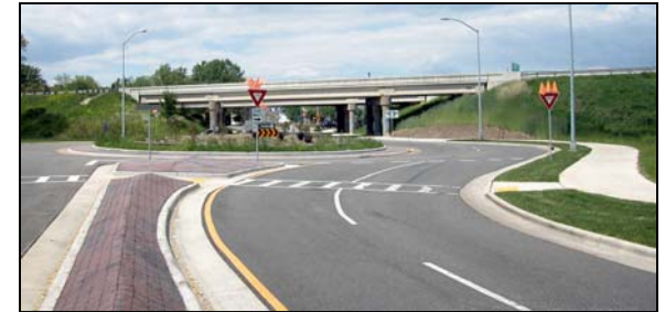
One of two roundabouts installed at the Swanton Road-Thompson Drive intersection.
